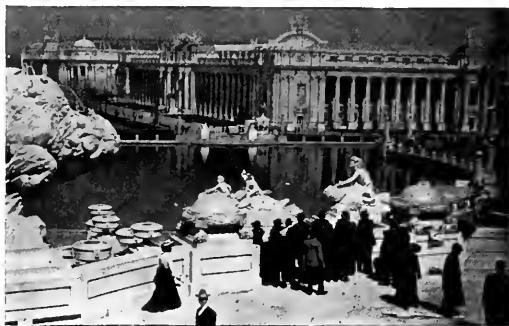
FIG. 17.—LOOKING TOWARD ELECTRICITY BUILDING.
